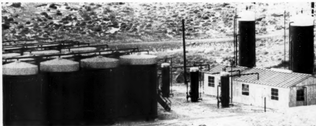
Sussex Unit "A" production scene, showing central separation and tank batteries for separate handling of Sussex, Shannon, and Lakota oils, left.
